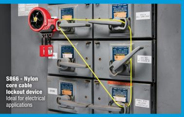
and hasps to secure the device during lockout
