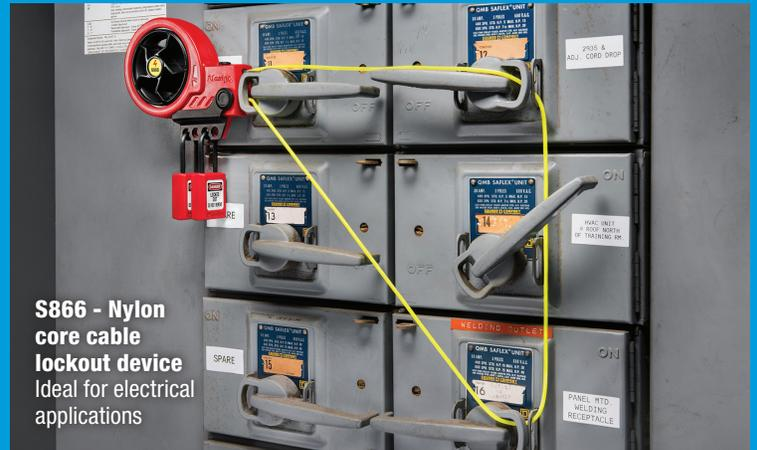
**S866 - Nylon core cable lockout device**
